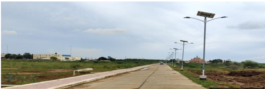
Solar Lights at the Entrance Road to VSU
