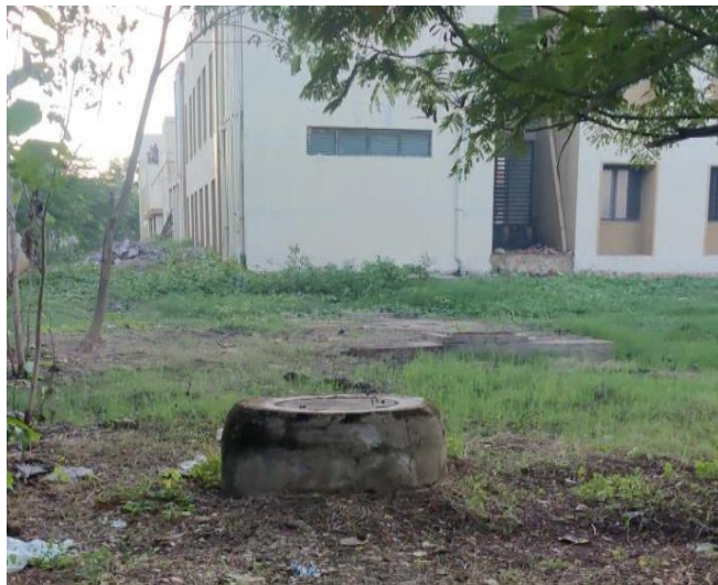
Underground drainage system for disposing grey water into soak pits
