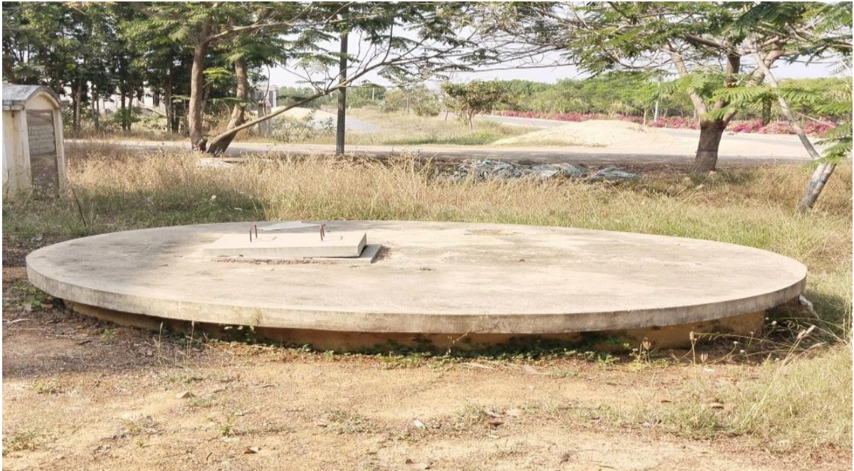
Rain water collecting tanks
