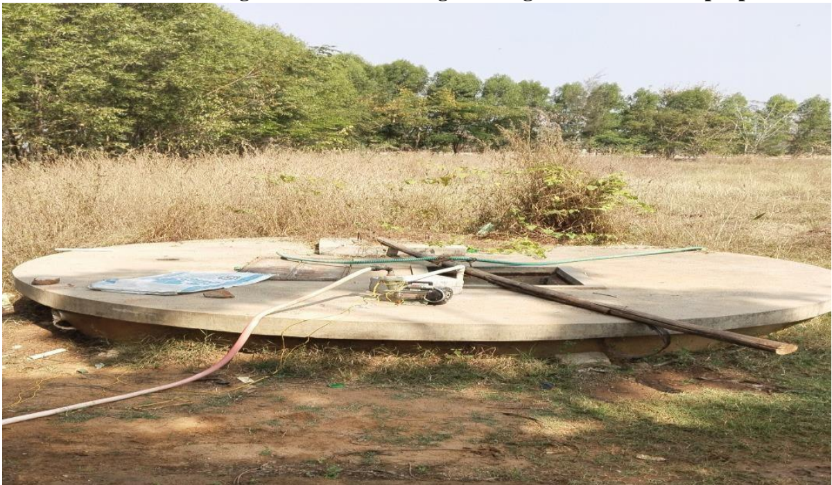
Rain water collecting tanks and used for gardening and construction purposes
