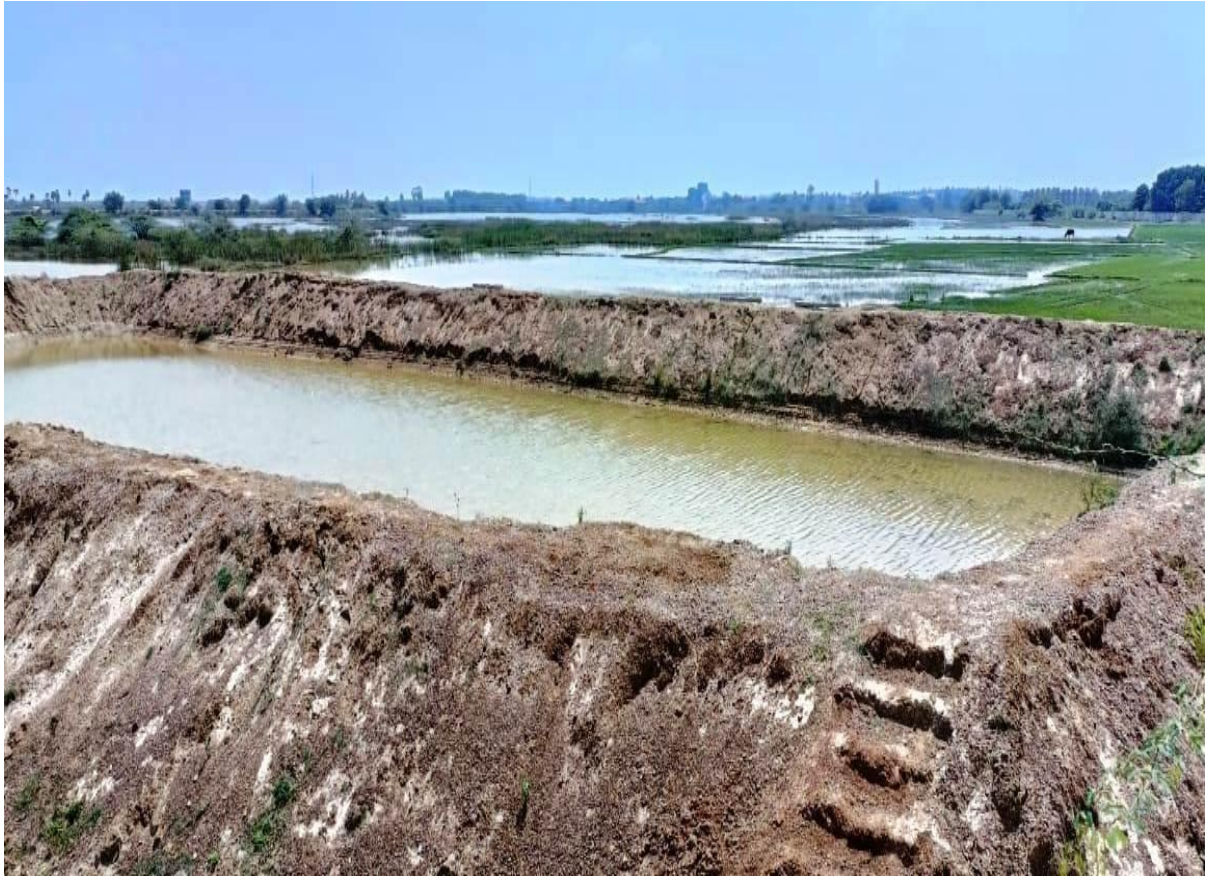
New pond constructed beside the tank for aqua research purpose
