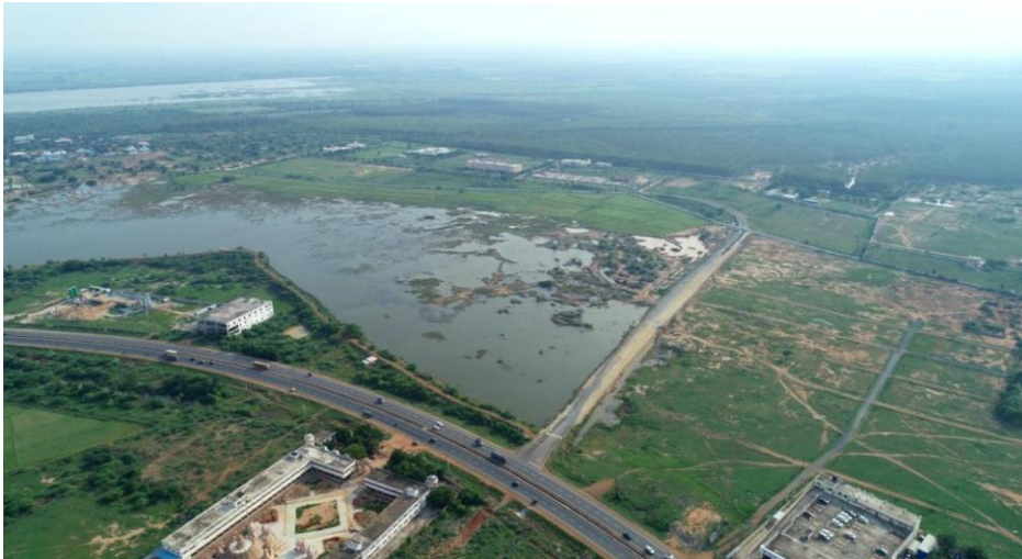
Large water tank near to University Main campus, Nellore
