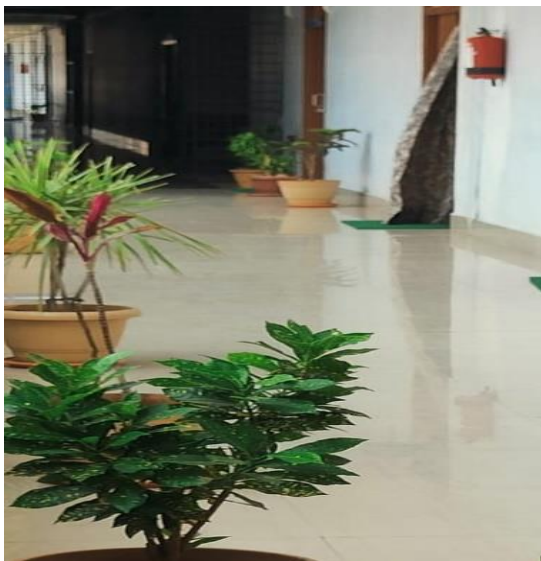
Fire safety at AD Building first floor
